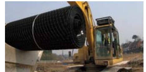
TriAx geogrid can be handled by machine or carried by two men.
