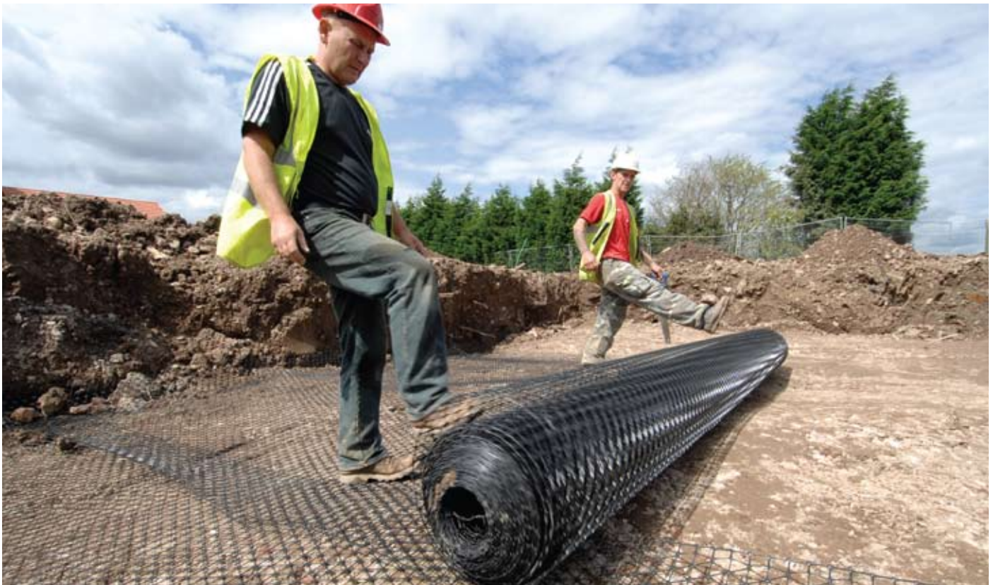
TriAx gives improved aggregate confinement and interaction, leading to improved structural performance of the mechanical stabilised layer.
