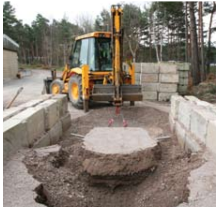
Excavation of TriAx for installation damage assessment at TRL.
