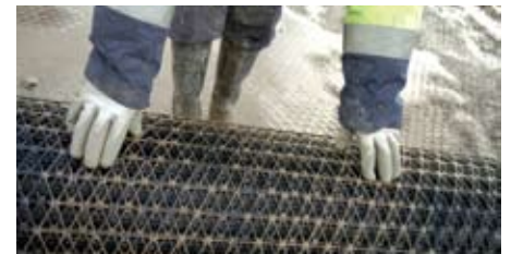
TriAx geogrid unrolled on site.
